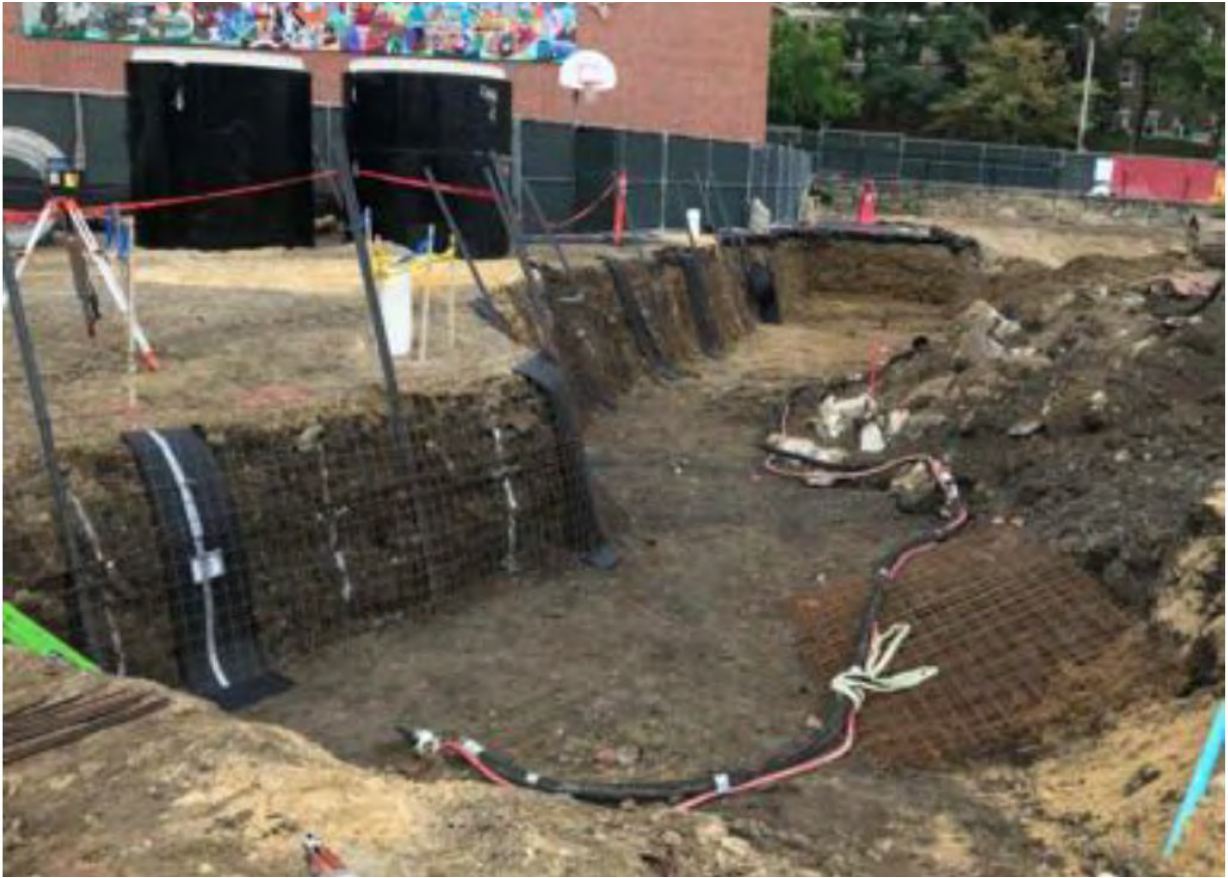
Prep for Shotcrete – 9/22/21
