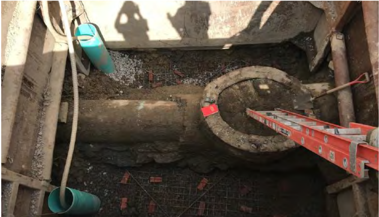
Rebar at Culvert Ready for Concrete – 9/3/21
