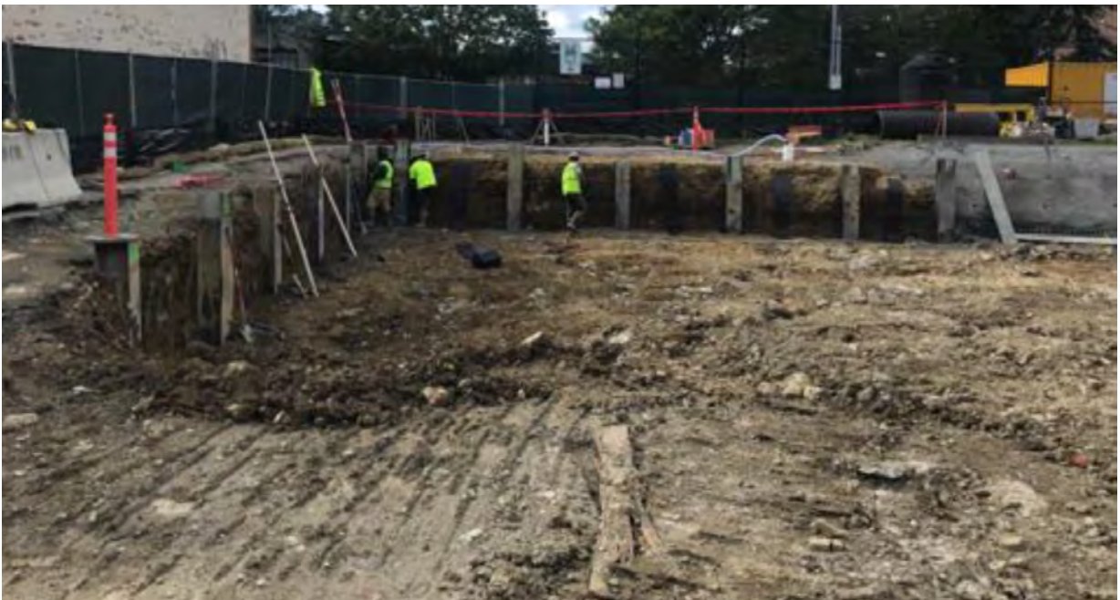
SOE Prep at Soldier Piles – 9/30/21
