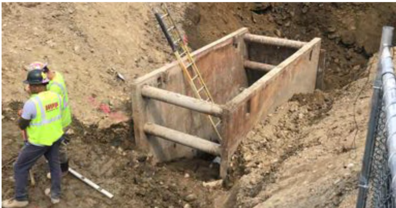
Excavation and Setting Pipe at South Side of Site – 9/15/21
